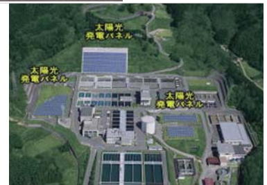
■ Gose Water Treatment Plant (Nara Prefecture)
