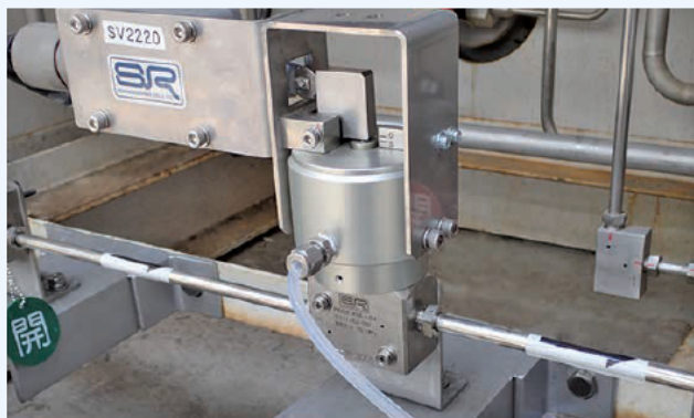
▲50MPa automatic hydrogen gas valve (installed at Toho Gas Co., Ltd.)
