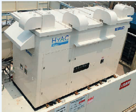
▲ Compressor for stationary hydrogen station "HyAC series"
