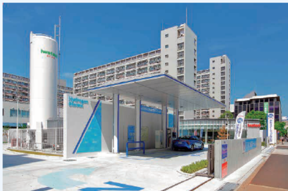
▲ Iwatani hydrogen station in Morinomiya, Osaka
