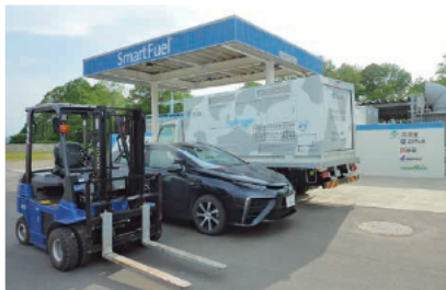
Hydrogen station on Shioikai Hydrogen Farm
