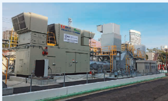
▲ Hydrogen gas turbine cogeneration system (Kobe Port Island) NEDO demonstration project: "Smart Community Technology Development Project Utilizing Hydrogen Cogeneration Systems" (FY2015 to FY2018) "Development and Demonstration Project for Dry Low-NOx Hydrogen-Fueled Gas Turbine Combustion Technology" (FY2019 to FY2020)
