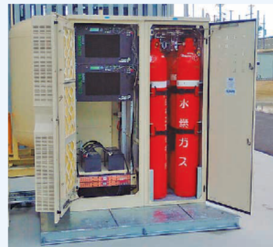
▲ Fuel cell system that can be utilized as an emergency backup power source without excess or deficiency by modularization of the power generation stack
