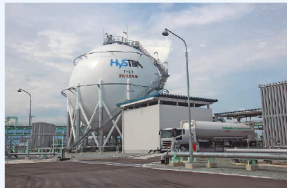
▲ Demonstration liquefied hydrogen storage and unloading facility constructed on Kobe AirPort Island
