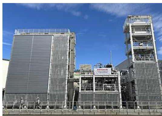
The facilities consist of two types of equipment: direct air capture equipment (on the left in the photo) that captures CO 2 from the atmosphere and post-combustion capture equipment (on the right in the photo) that captures CO 2 from the exhaust gases of the factory's in-house power generation equipment.
