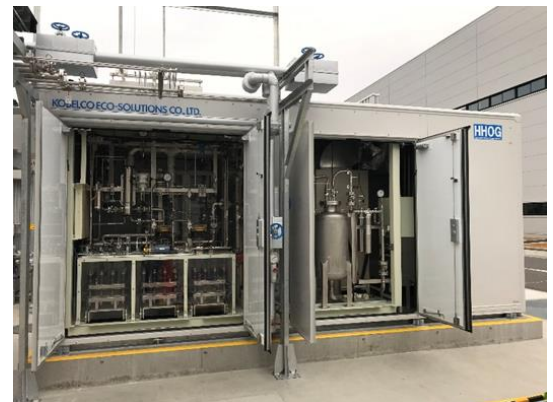
Water electrolysis-based high-purity hydrogen and oxygen generator Skid-mounted type: 20 Nm 3 /h
