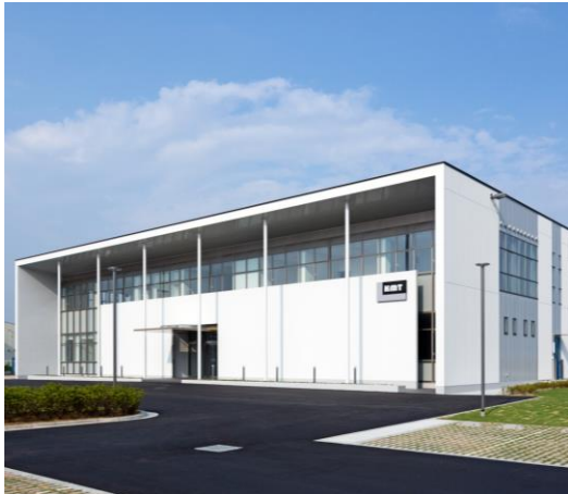
<Kobe Material Testing Laboratory – Head Office> The facility is equipped as an advanced materials evaluation center, including a dedicated area specifically designed for high-pressure hydrogen testing.
