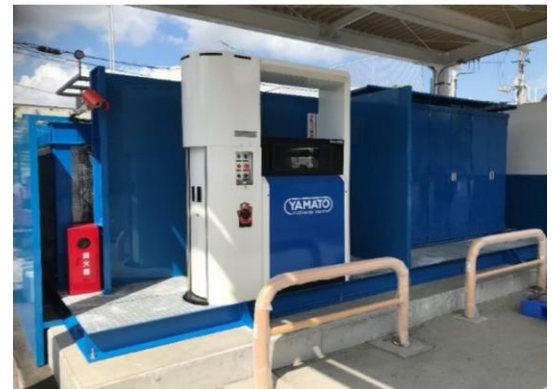
Packaged hydrogen station for 70 MPa FCVs and 35 MPa FCFLs
