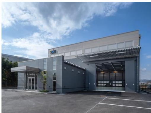
Thermal Technology Laboratory (Ikoma District, Nara Prefecture)
