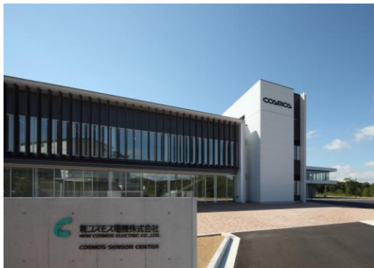
Gas sensor research facility "Cosmos Sensor Center"
