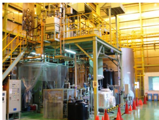
Demonstration equipment for aluminum dross processing
