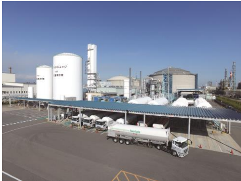
Hydro Edge, Japan's largest liquefied hydrogen production plant
