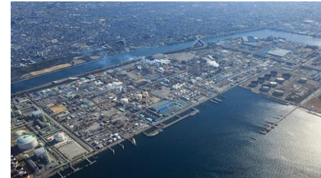
Hydrogen/Ammonia Supply Chain construction
